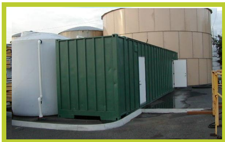
Pictured: Washougal, WA- The ElectroPulse (EC) System used here successfully removed contaminants from stormwater.
